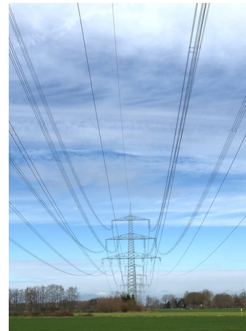
Transmission power line (ref: DLR)
